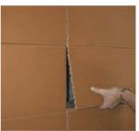
Push two panels arranged above the panel to be replaced upward, press panel upward, remove it and replace it by a new panel.
