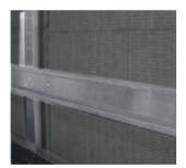
Connect horizontal system rails to pre-mounted vertical substructure by means of approved fastening means.
