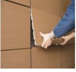
Insert 2 mm thick sheet metal in horizontal joint, press upward and remove panel (possibly push panels on top of it upward in addition). Hang the panel in the system rail from top towards the bottom.
