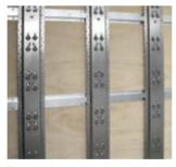
Exactly align the profiles, observe grid distance
