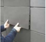
Insert 2 mm thick sheet metal in horizontal joint, press upward and remove panel (possibly push panels on top of it upward in addition). Hang the panel in the system rail from top towards the bottom.
