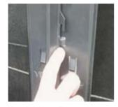
Hang in joint profile or insert spacer
