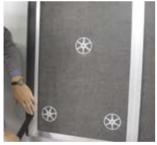
Apply joint tape on vertical bearing
