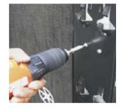
Fasten system rail with screws\* or rivets\*\* (only use approved fastening means - it is absolutely necessary to fix the rail under each fastening hook!)
