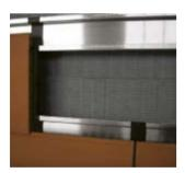
Hang panels with pre-mounted adapters in the horizontal rails. Cover horizontal profile at the joint with black joint tape or black paint.
