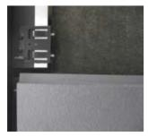
Profile butt joint with edge-clamps 682 and 683
